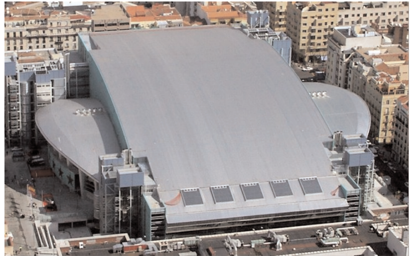
Figura 2. Vista general. Figure 2. General view.
