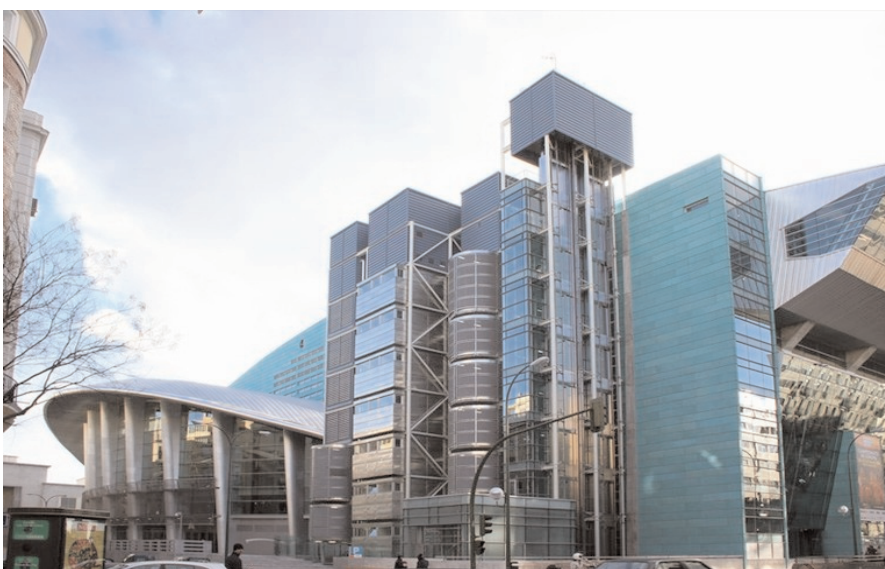
Fig. 18. Torres de Servicios. Figure 18. Service tower.
